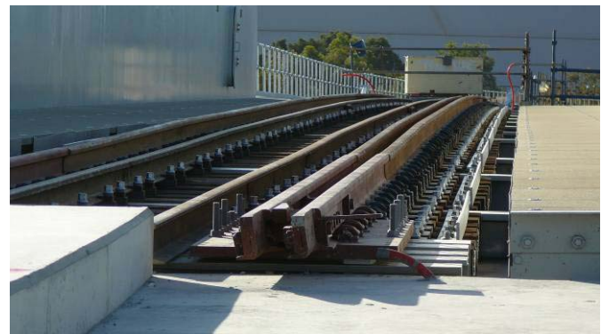
Photo – View of Vertical Curve on Lift Up Span
