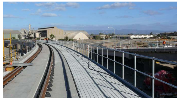
Photo – View Port Adelaide Side of Bridge
