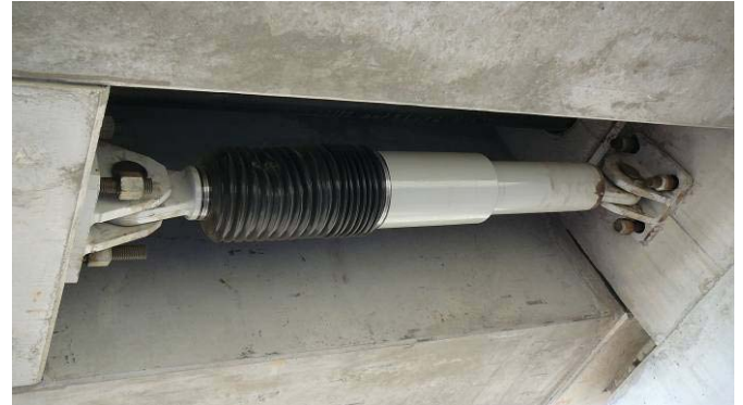
Photo – View of Lock-Up Device
