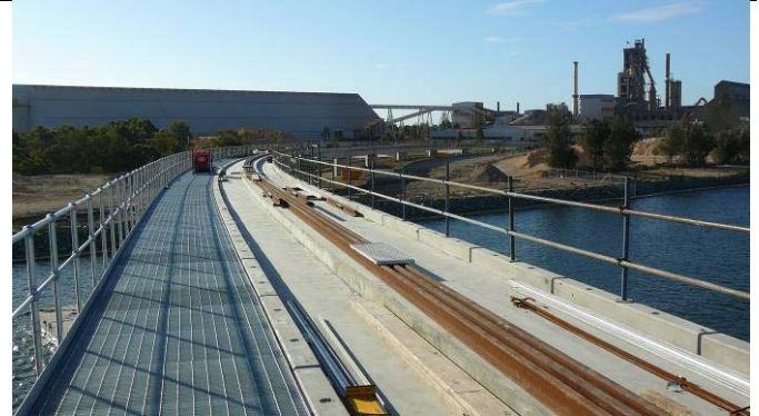
Photo – View of Outer Harbor Side of Bridge
