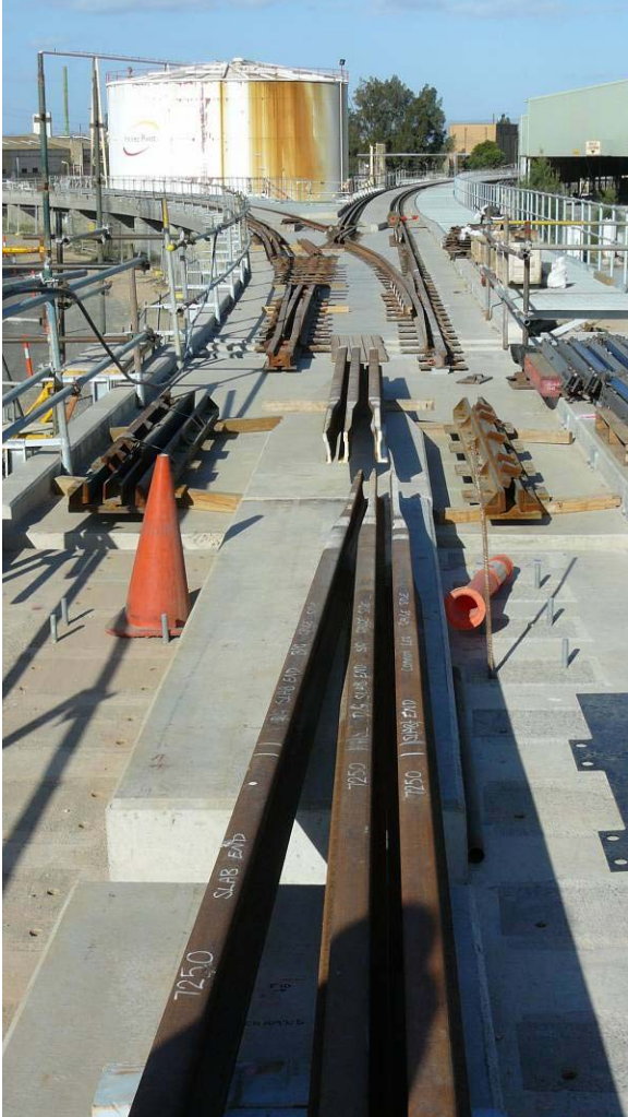
Photo – View of Port Flat turnout and Expansion Rails
