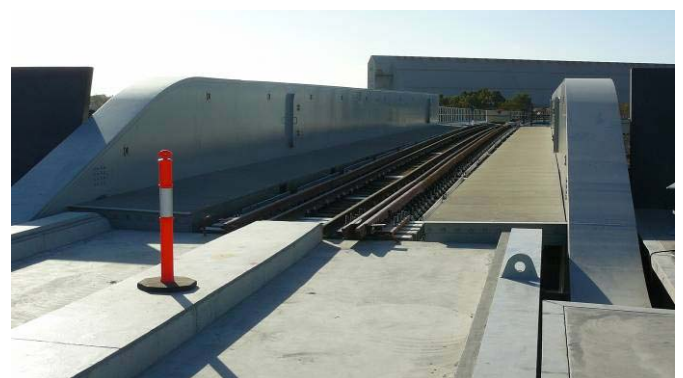
Photo – View of Inside of Lift Up Span
