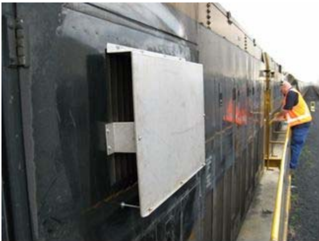
Photo 7 – 92 Class Locomotive Air Intake Deflectors
