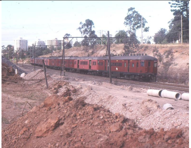
Parramatta Park – dive under construction
