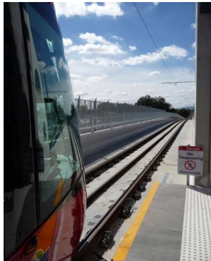
Tram on the South Road overpass
