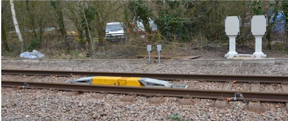
Figure 4 Trial installation of LCWS version 1.1 at Maltings, UK
