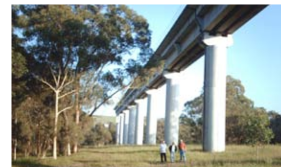
The Nepean River approach viaducts constructed in 1985 for the Maldon Port Kembla Railway Photo: Leon Oberg/Track and Signal
