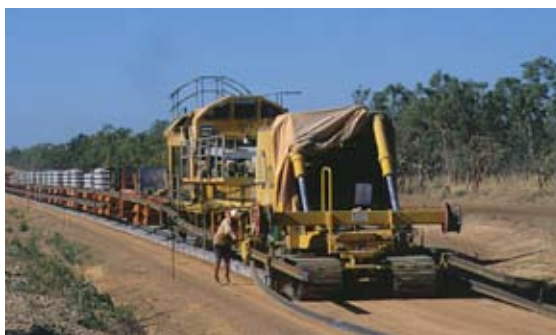
Tracklaying on the Alice Springs – Darwin railway. Photo: Mark Carter
