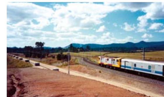
A Queensland Main Line Upgrade (Tandur Traveston deviation). Such mainline track straightening is recommended for New South Wales. Photo: Philip Laird
