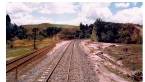
A North Island Main Trunk small deviation slices through a hill Photo: Philip Laird
