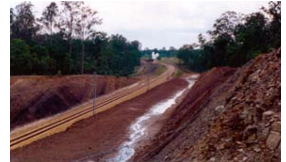
The old meets the new. A 1995 Waltzing Matilda steam train seen on the then new Gunalda deviation in March 1995. This 8km deviation replaced 10 km of 'steam age' alignment and cut up to 8 minutes of transit time.
